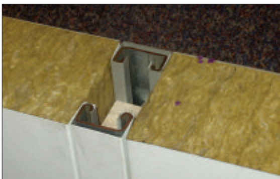
Figure 17: Insulated core panels – internal panel
