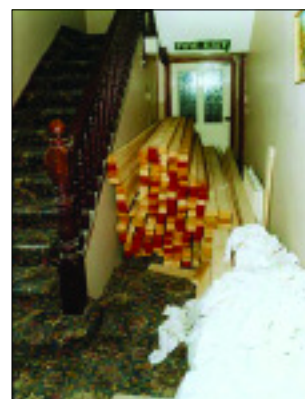
Figure 9: A blocked corridor with incorrect signage
